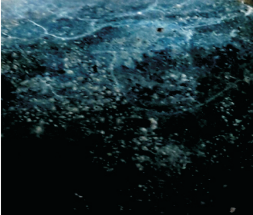
Figure 9- Material of pipe after exposure to water sample no-23
